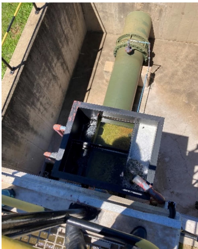
Figure 3-49: Inlet chemical dosing and flow splitting
