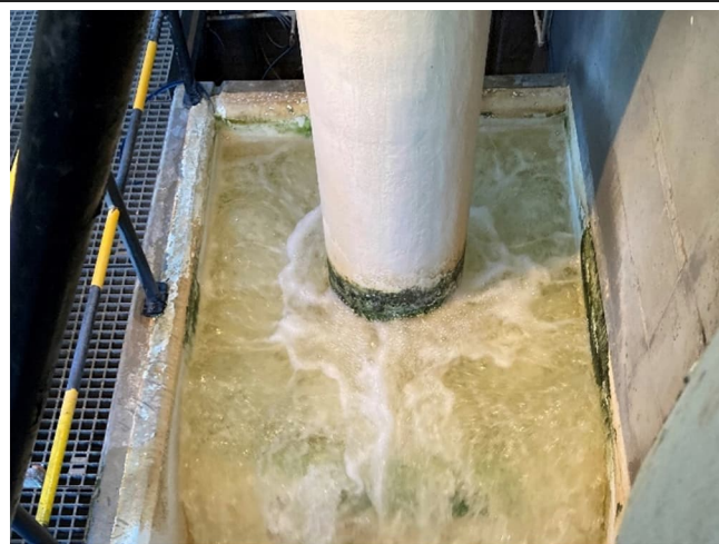
Figure 3-62: Filtered water inspection chamber (partialisation-siphon system over-aerating)
