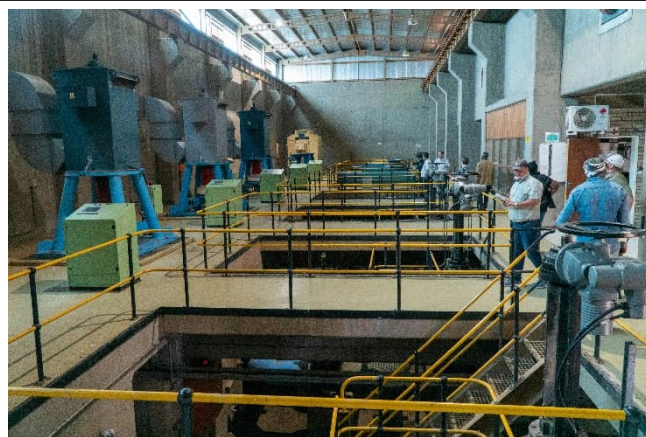
Figure 3-22: Six pump sets installed
