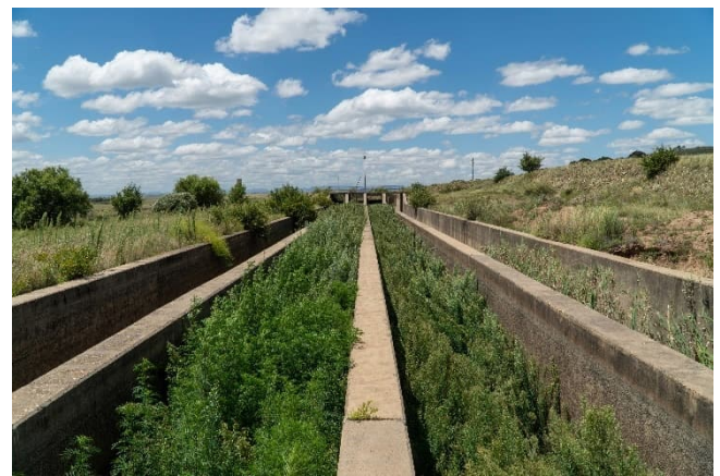
Figure 3-18: Overgrown and silted up channels
