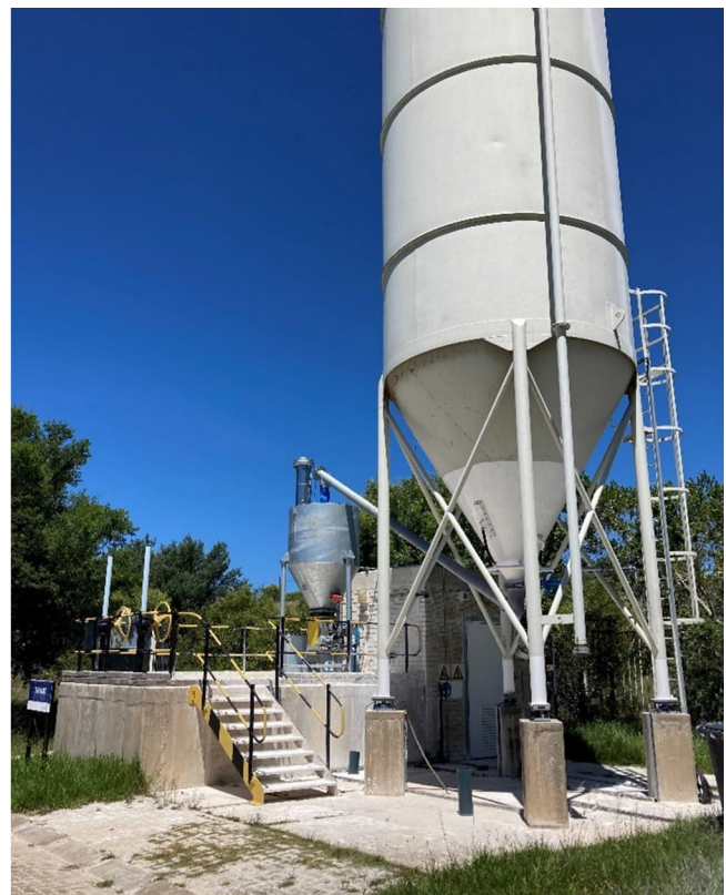
Figure 3-50: Lime dosing equipment
