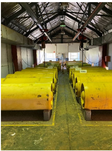
Figure 3-65: Chlorine drums
