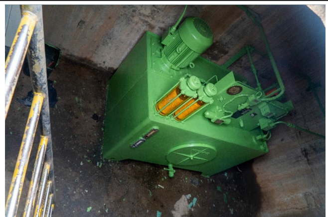
Figure 3-34: Newly painted hydraulic power pack
