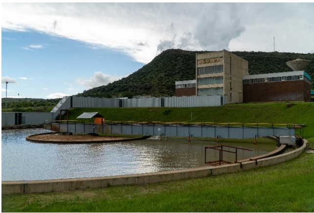
Figure 3-41: Primary sedimentation - clariflocculator
