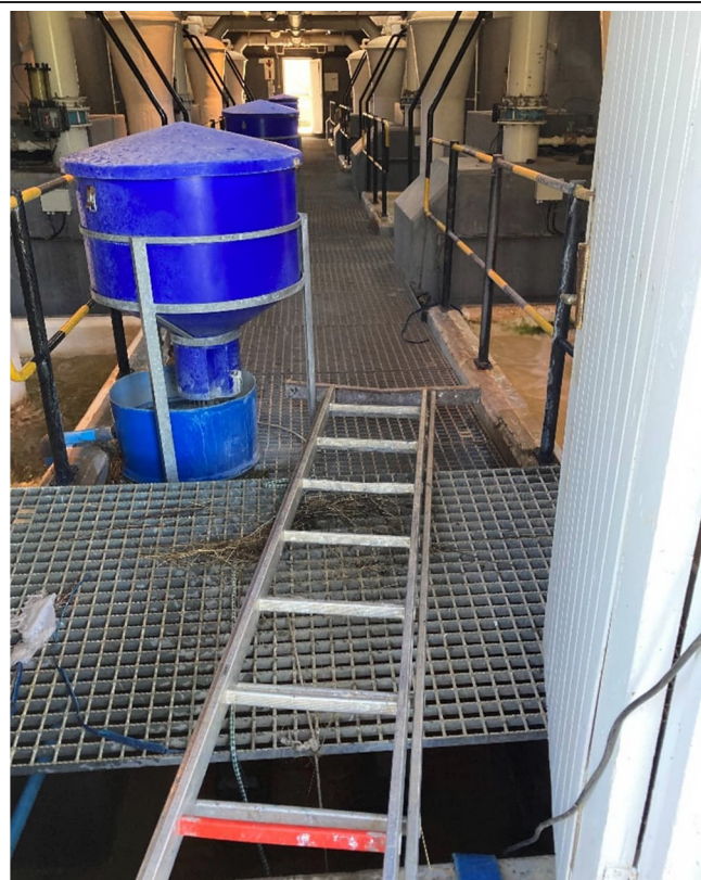
Figure 3-60: Lower filter gallery (unsafe access)
