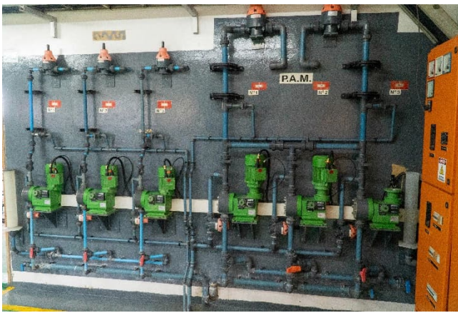
Figure 3-39: Coagulant dosing pumps
