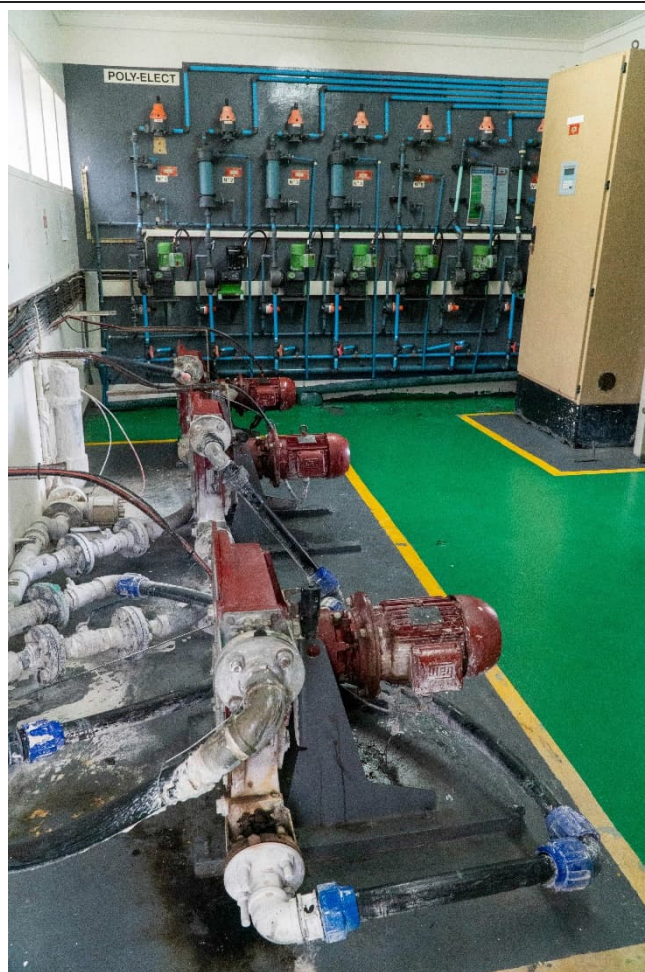
Figure 3-38: Lime slurry dosing pumps
