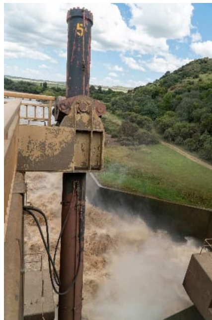
Figure 3-32: Sluice gate 5 hydraulic piston
