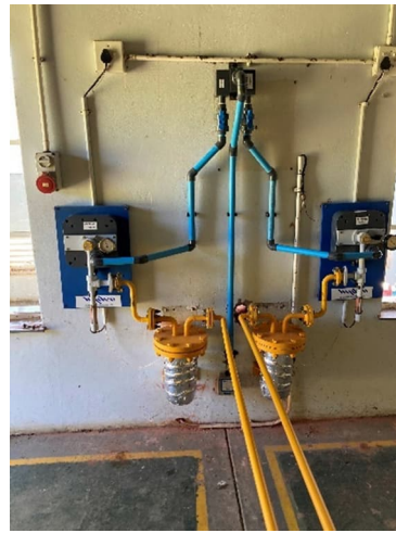
Figure 3-64: Chlorine dosing equipment
