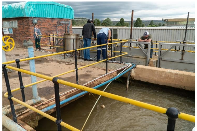
Figure 3-42: Agitators and secondary dosing point
