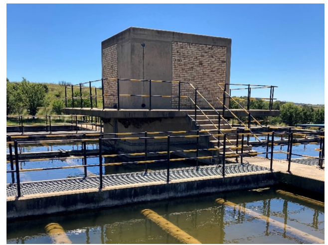
Figure 3-54: Pulsator vacuum control building
