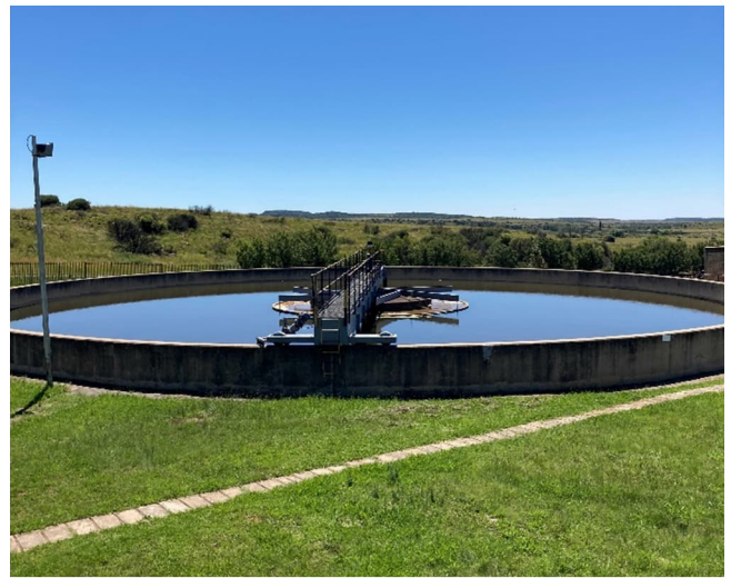
Figure 3-52: Turbo-circulator clarifier
