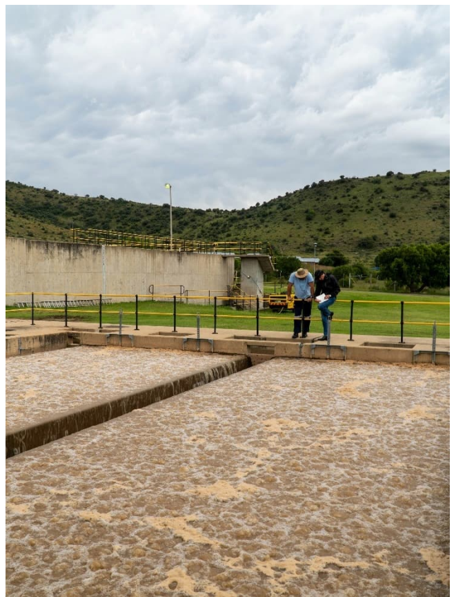
Figure 3-44: Filters backwashing
