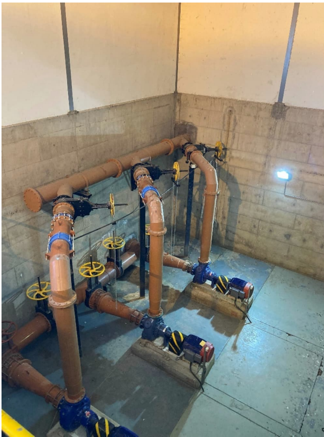
Figure 3-67: Residuals pump station
