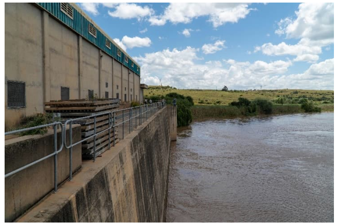
Figure 3-26: Abstraction inlet screening wall
