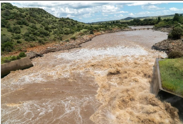
Figure 3-33: Evidence of downstream scouring and debris
