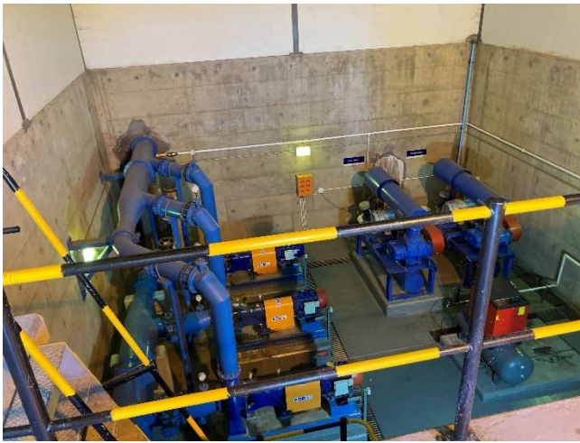
Figure 3-63: Filter backwash pumps and air scour blowers
