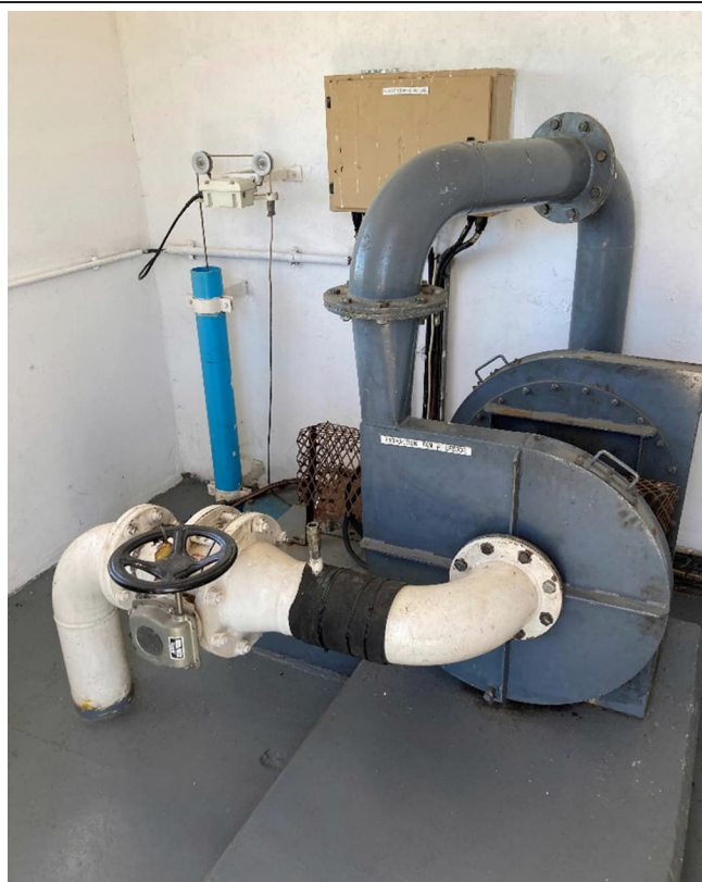
Figure 3-55: Pulsator vacuum pump (not operable)
