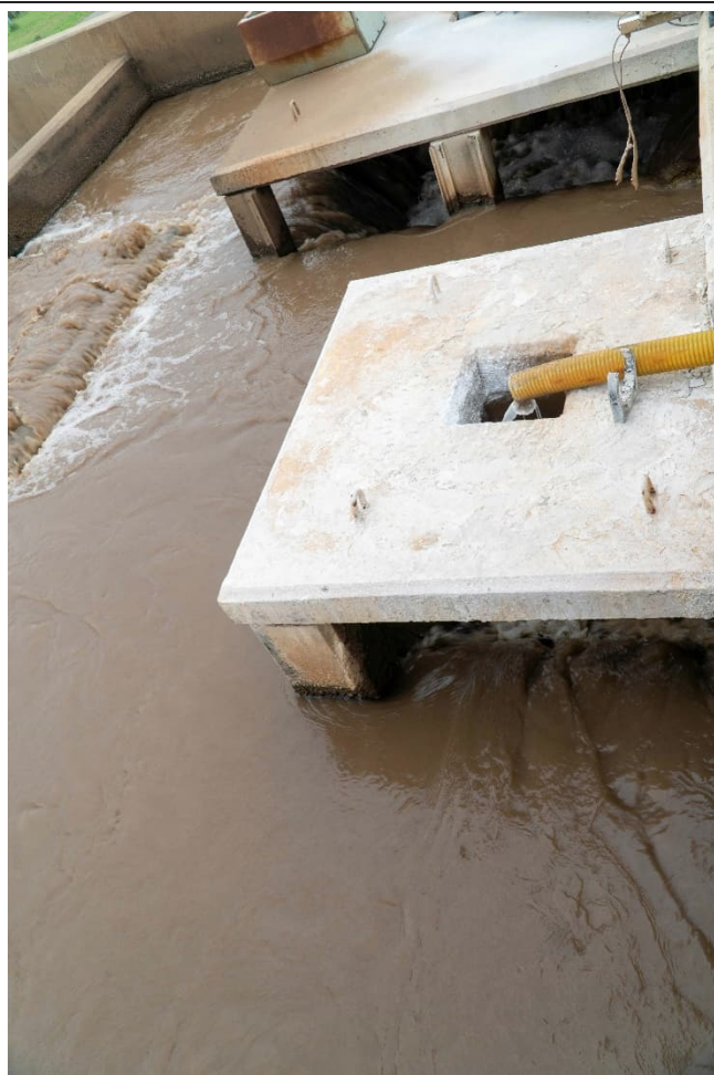
Figure 3-37: Lime dosing
