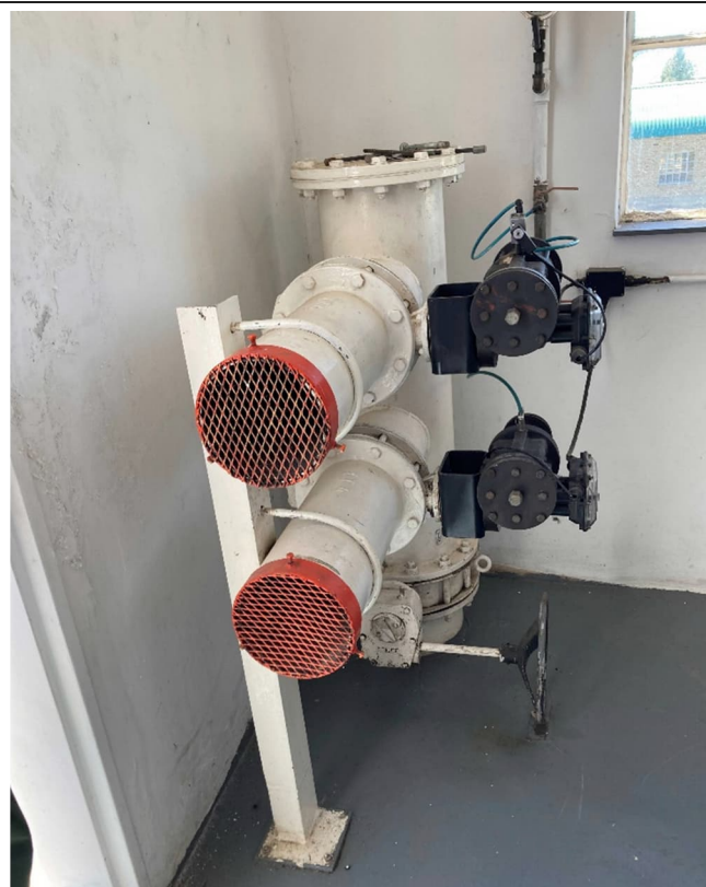
Figure 3-56: Pulsator vacuum control equipment (not operable)
