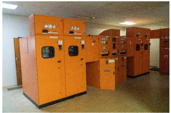
Figure 3-6: MCC in Control Room
