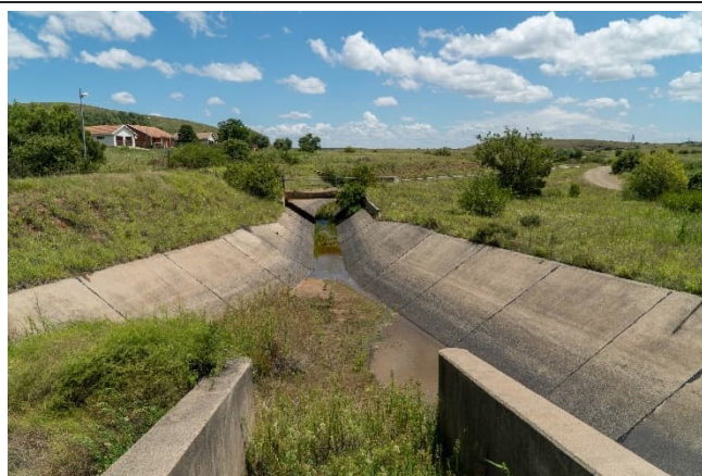
Figure 3-19: Downstream channel also overgrown
