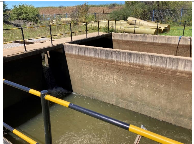
Figure 3-66: Residuals holding tanks
