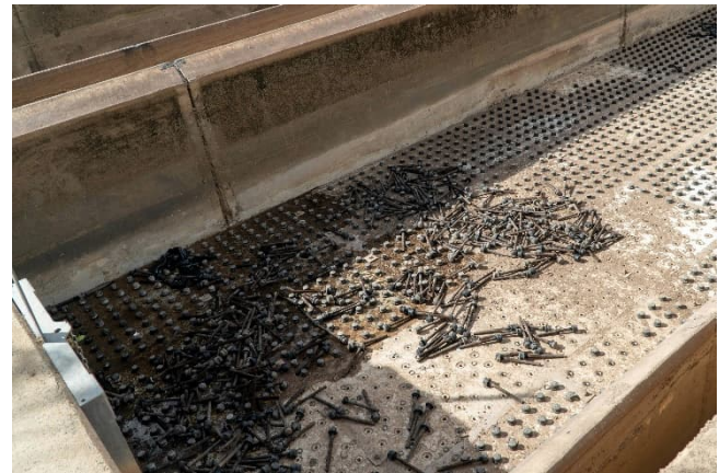
Figure 3-48: Filtration nozzles being replaced
