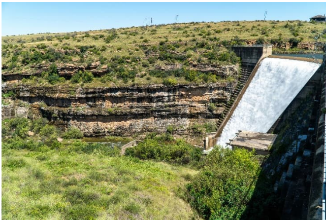
Figure 3-11: Water seeping through dam wall on right side of image
