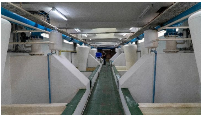
Figure 3-45: Filter lower gallery and partialisation / siphon system
