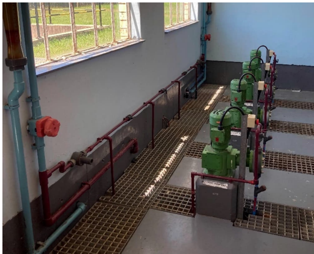
Figure 3-51: Coagulant dosing equipment
