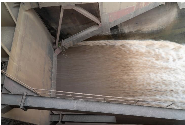
Figure 3-31: Sluice Gate 5 open
