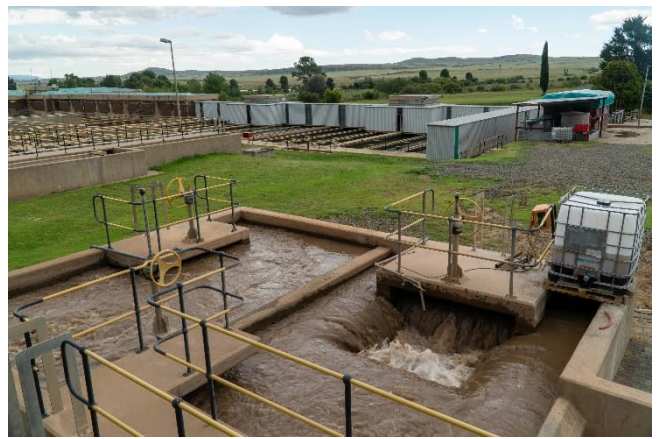
Figure 3-40: Inlet mixing and flow splitting
