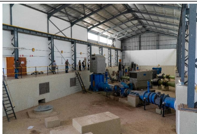
Figure 3-2: Novo pump sets with one open pump bay
