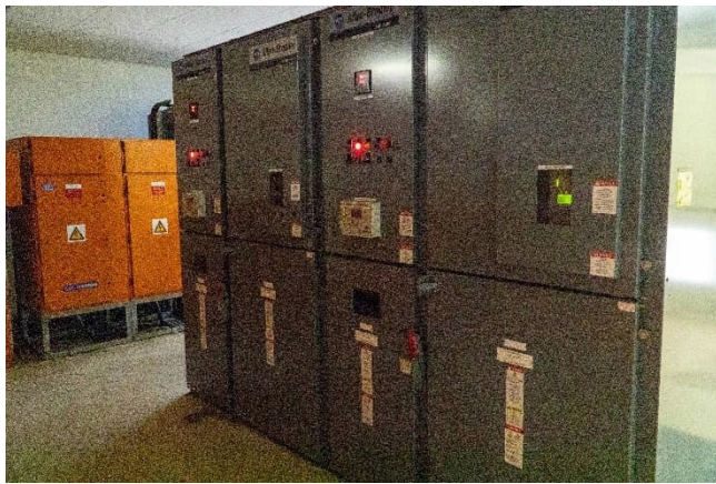
Figure 3-5: MCC in Control Room
