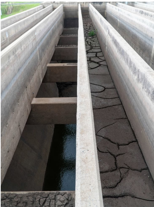
Figure 3-43: Primary sedimentation – horizontal flow system
