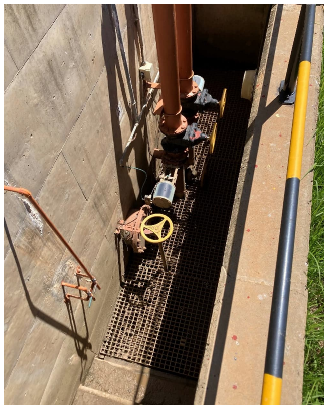
Figure 3-57: Pulsator de-sludge valves (actuators not operable)
