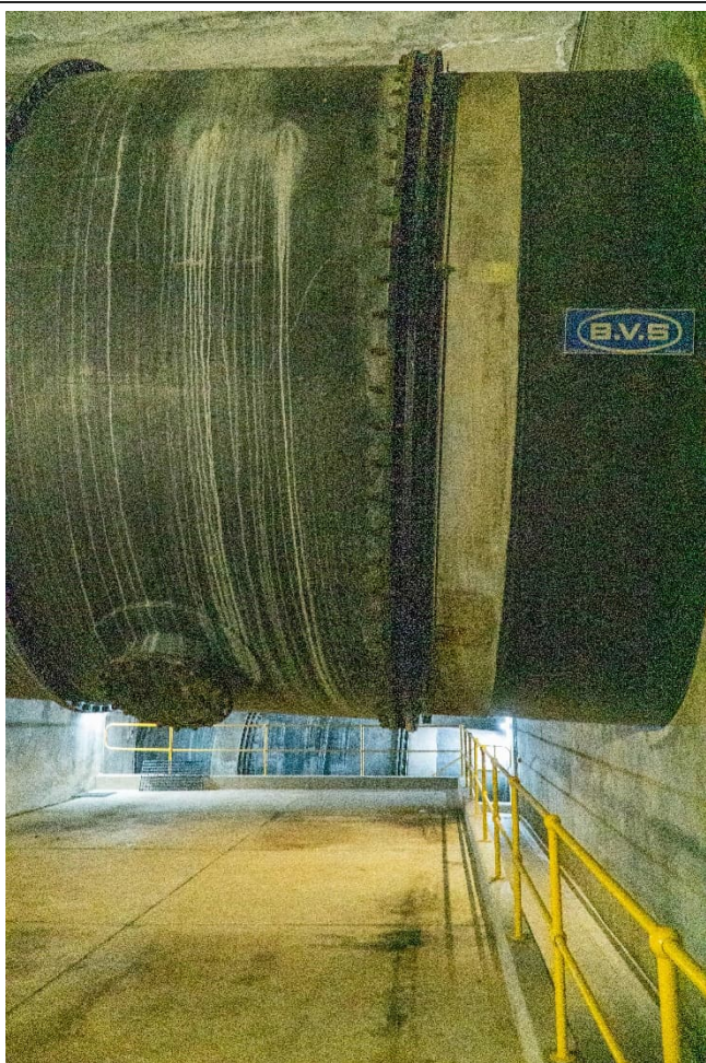
Figure 3-73: One of the existing 2.1m Ø pipes within the dam wall
