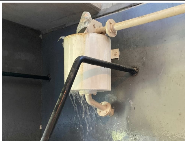
Figure 3-61: Filter float chamber overflowing
