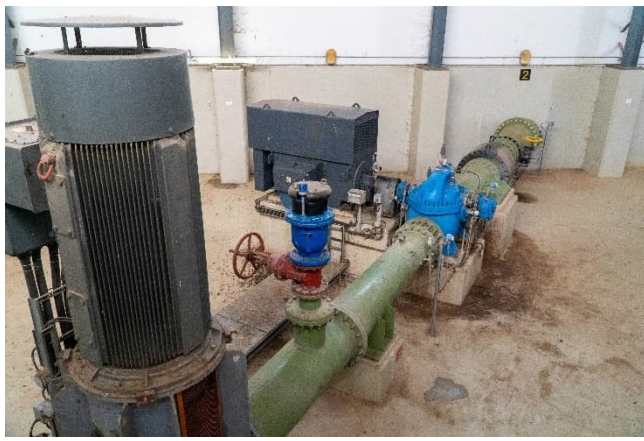
Figure 3-3: Original pump set
