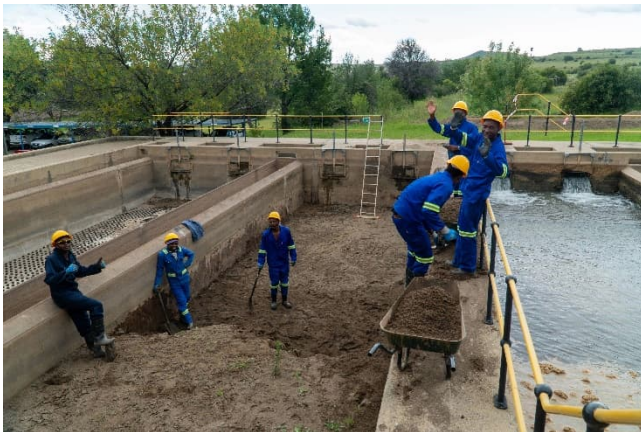
Figure 3-47: Refurbishment of filter under-drainage system in process
